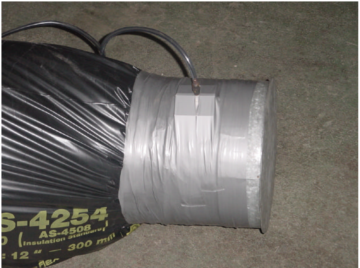
Figure 3: Pressure Measurement at Capped End
